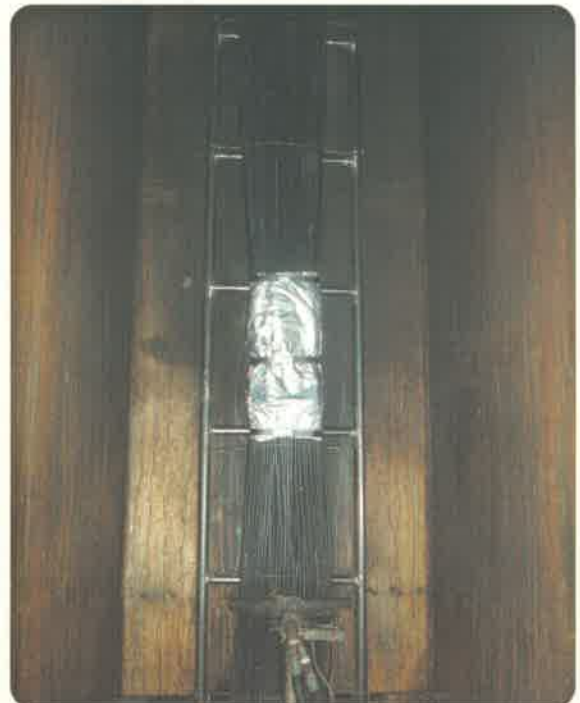
▲ Before Fire Test (Fire stop system A-119N)
