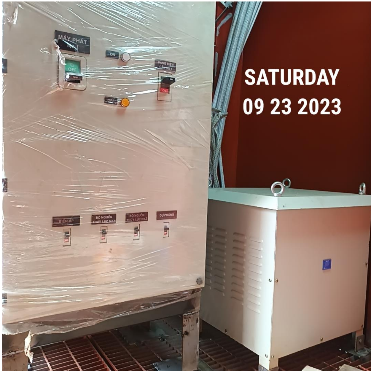
Manufacture of charging cabinets
