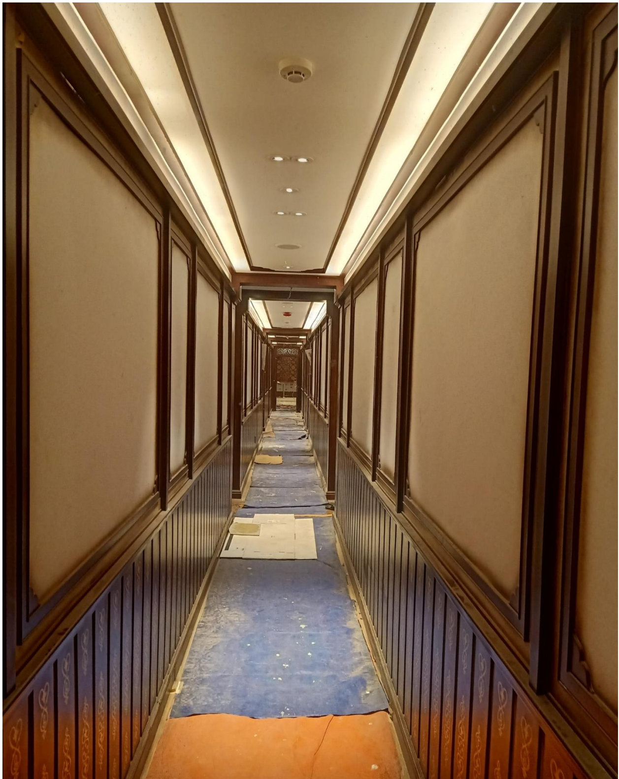
Installation of the entire lighting system for Ylang
