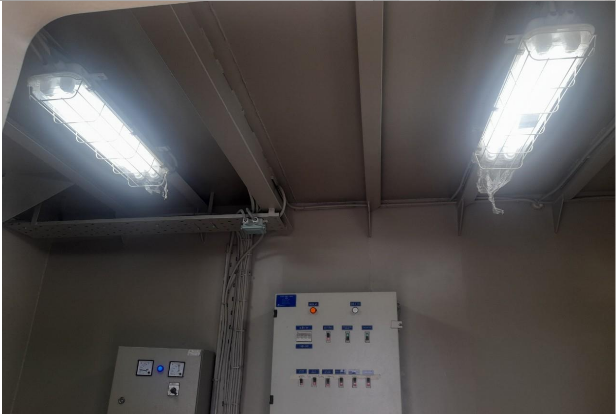
Installation of lighting system
