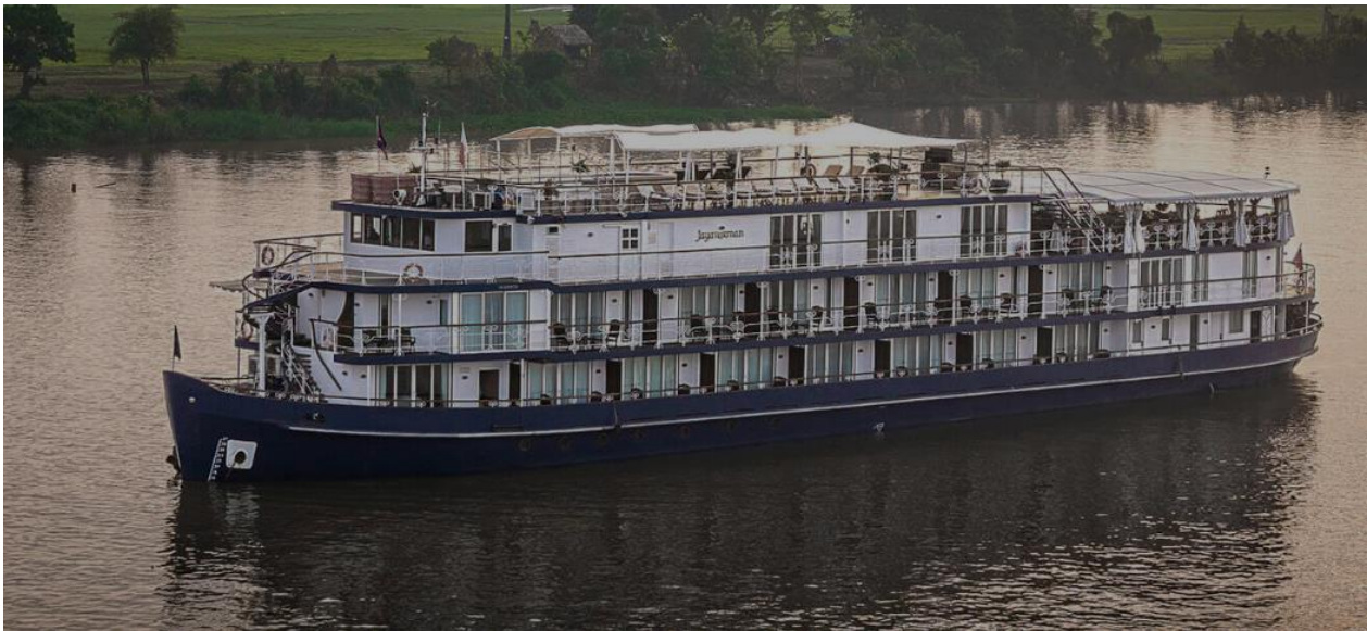
Supply and construction of the whole electrical system for JAYAVARMAN passenger vessel
