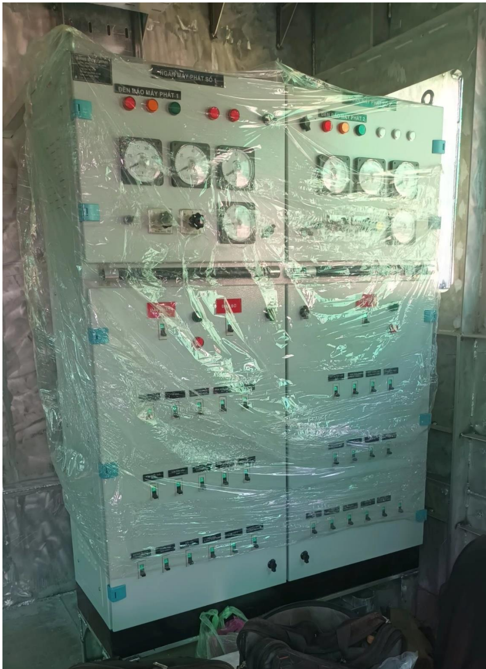
Manufacture electrical cabinets for tourist vessel
