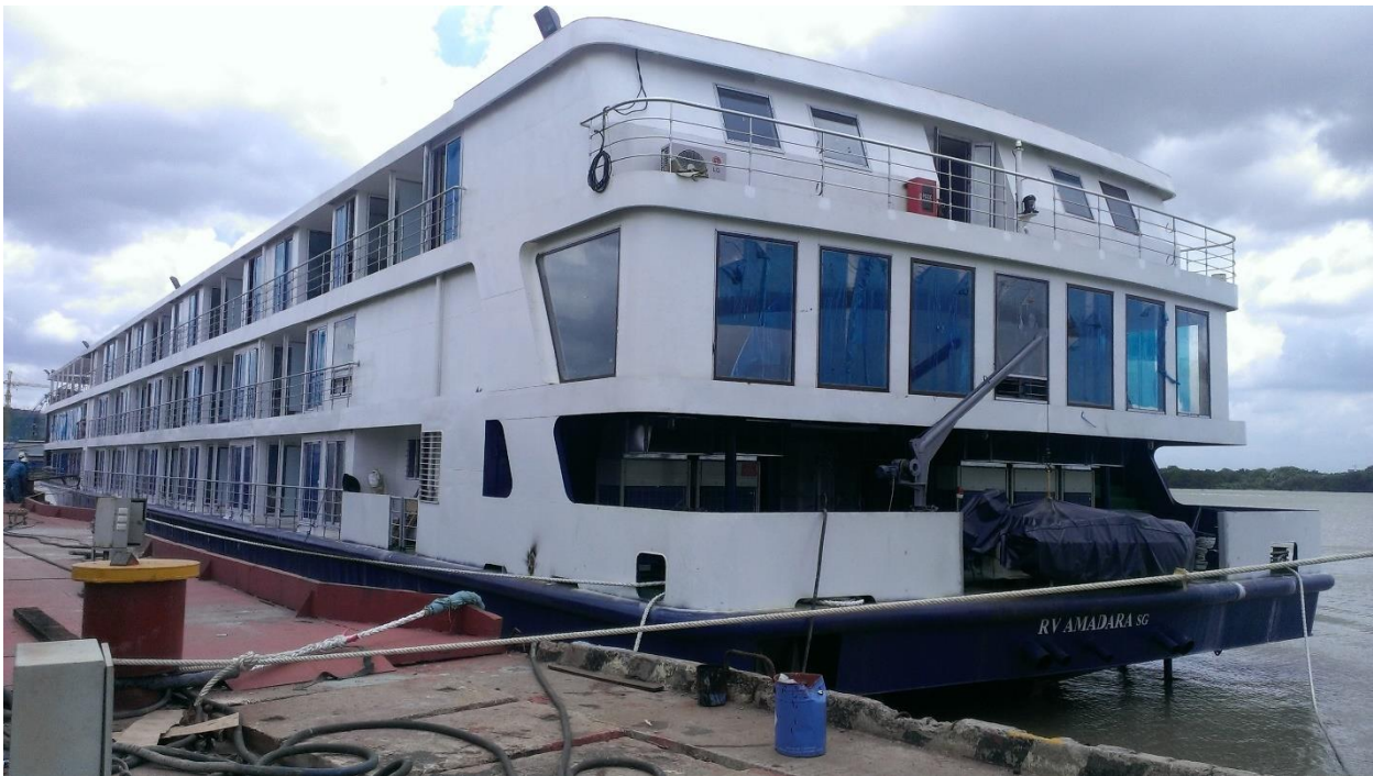
Construction of electrical system for RV AMADARA
